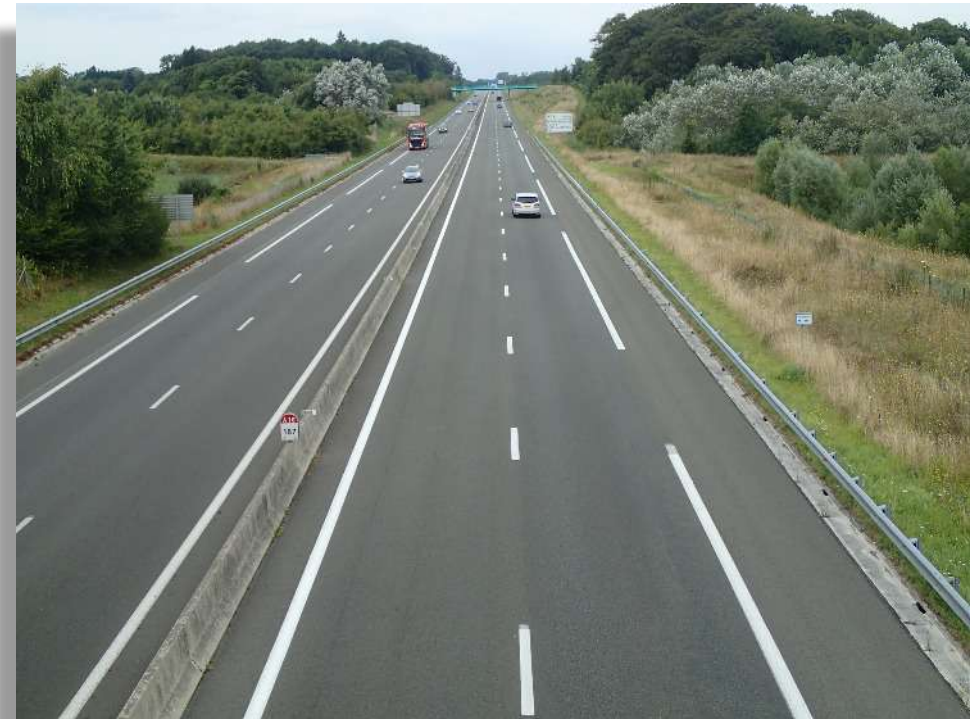
Autoroute A16 Forest-Montiers
